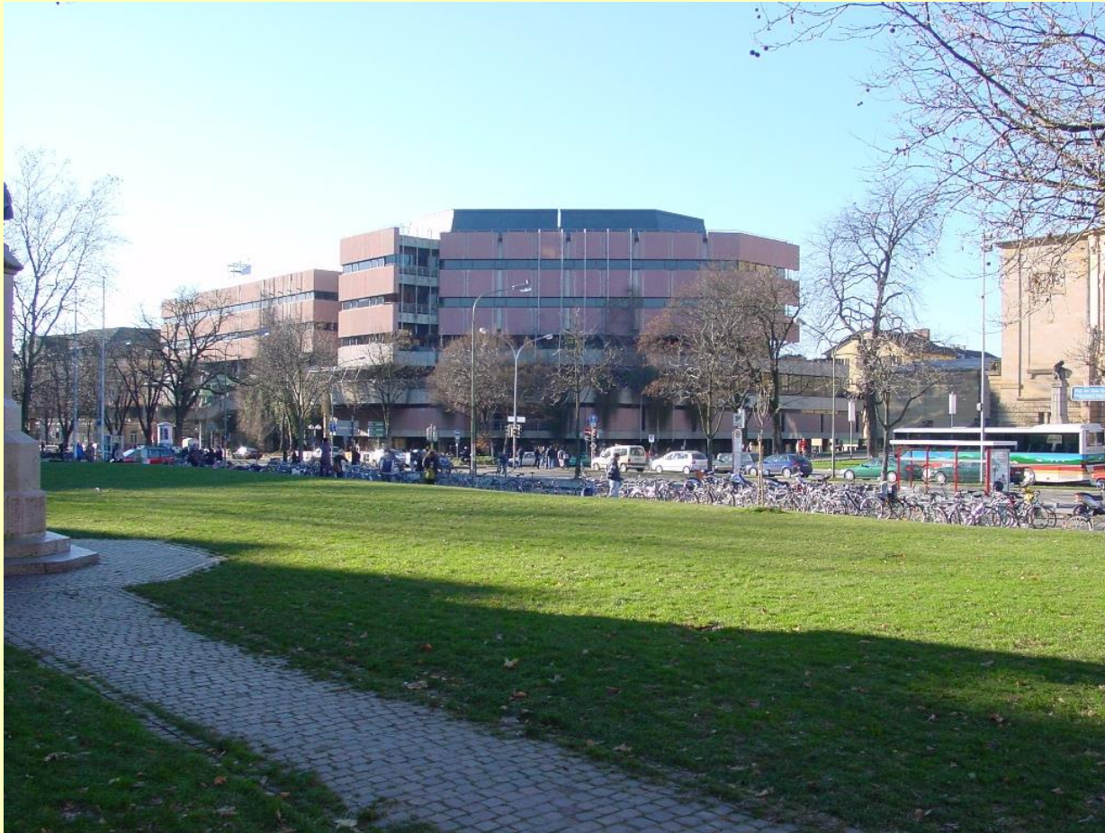
View Northeast – from the Place of the Old Synagoge
