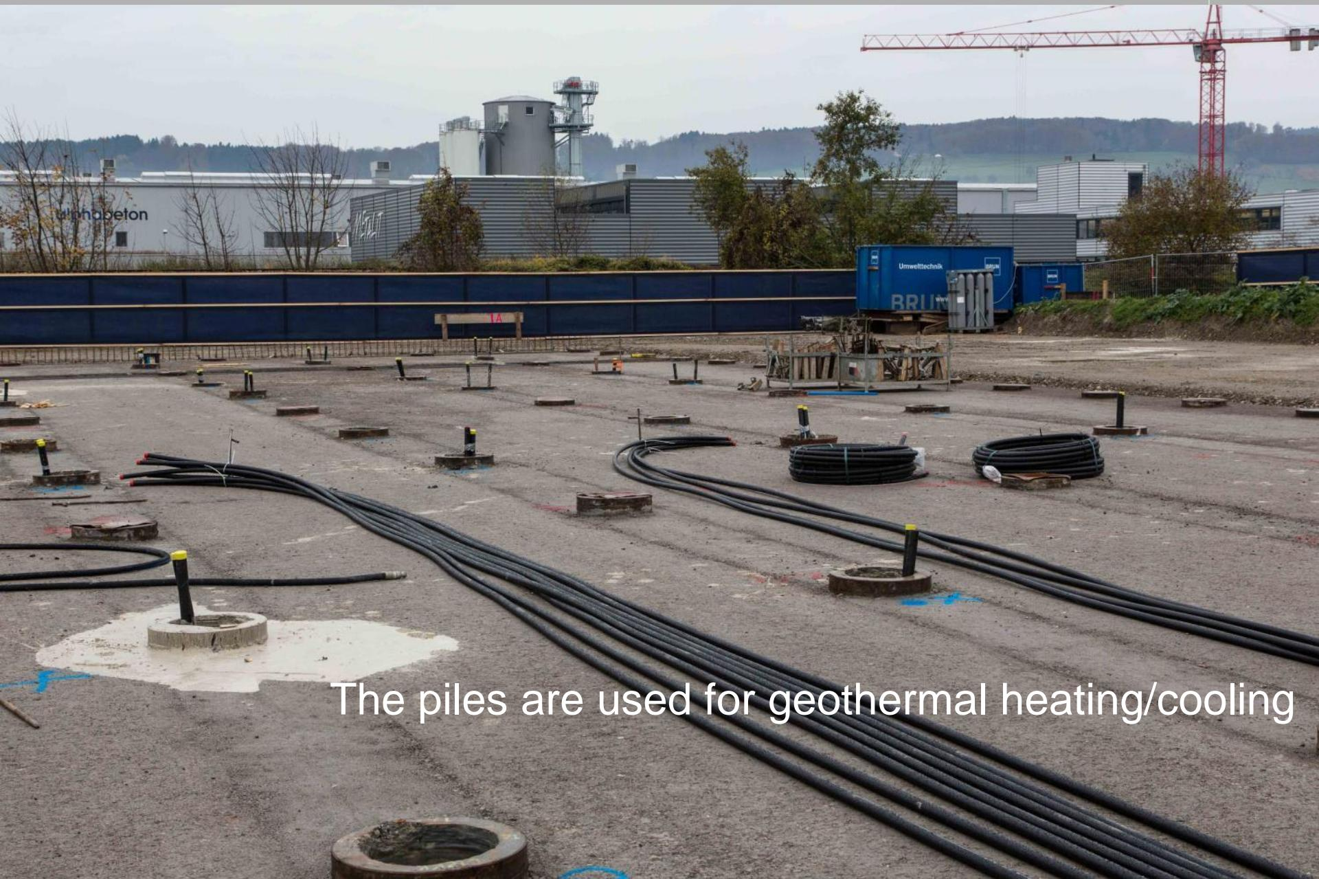
The piles are used for geothermal heating/cooling
